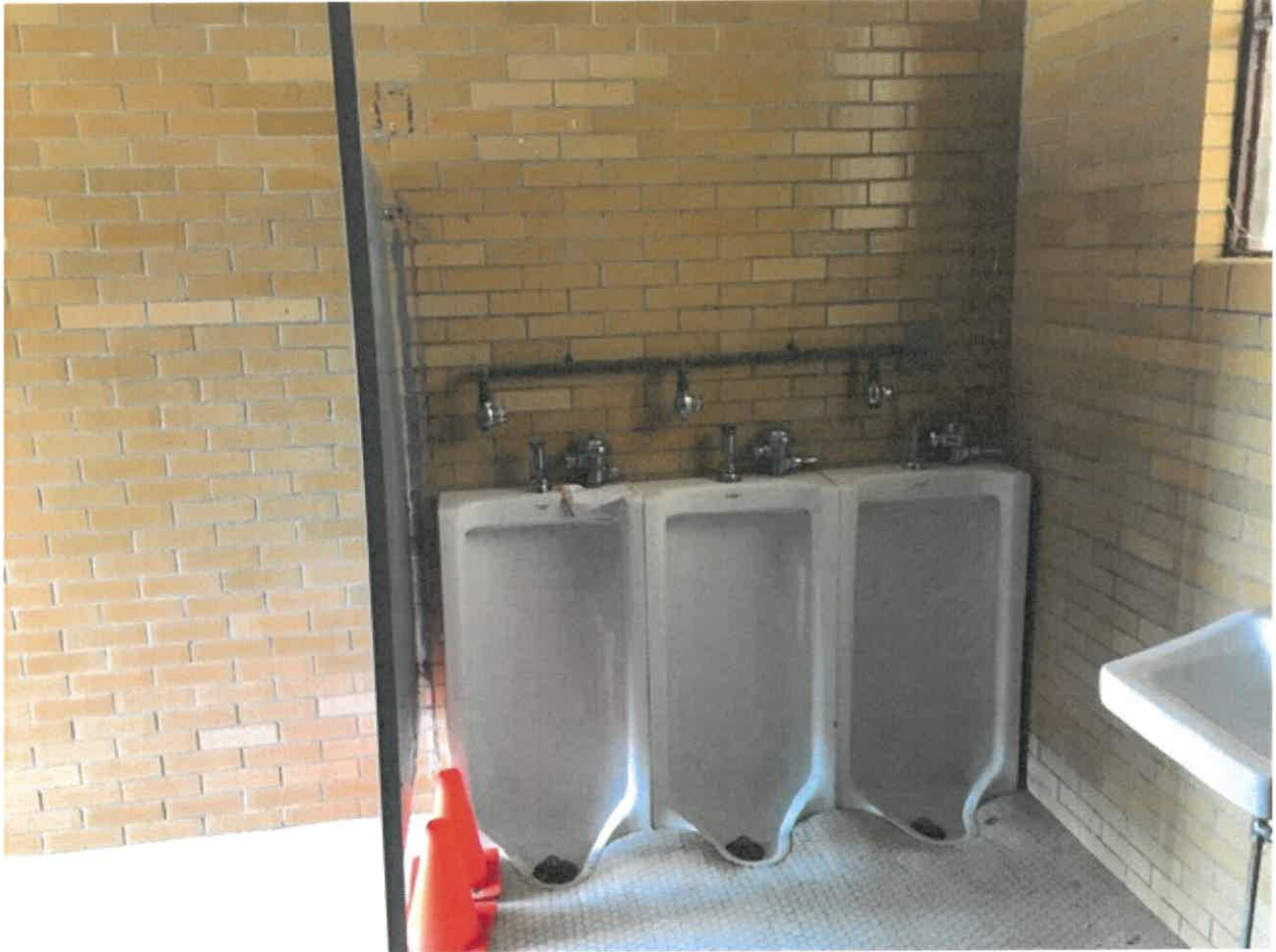
The existing urinals would remain.
