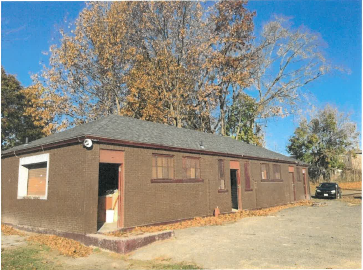
The Restroom / Storage Building at Deming Park.
