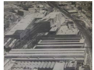
General Electric's transformer business boomed in Pittsfield during the middle decades of the 20th Century.
